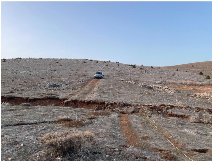
**Fig. 2 Surface ruptures caused by the 2023 Kahramanmaraş Earthquake Sequence.** Dirt roadway offset near the epicenter of the Ekinozu earthquake. Photo by Sinan Akciz, California State University, Fullerton.
