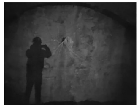
(b) Field blasting network
