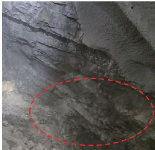
Figure 20. Effect of directional protection energy-gathered blasting.
