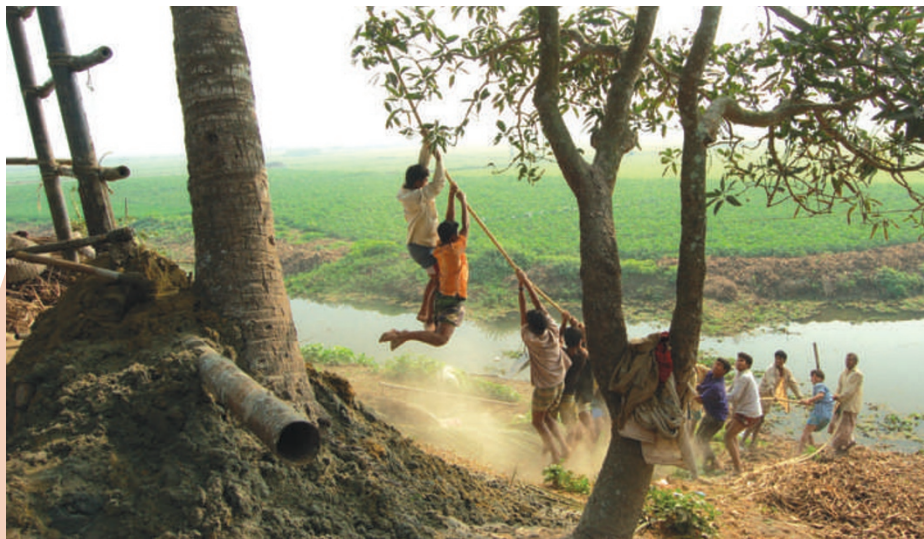
Villagers pulling a drill rod out of a newly drilled well, so that it can be replaced with PVC piping.
